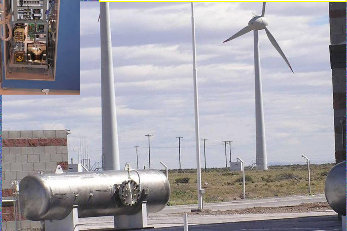
Stuart 5kW Electrolyzer & ITBA 6kW Electrolyzer • Production of Hydrogen from Wind-fed grid. • Experimental and research facilities • Uses: modified internal explosion vehicles and small fuel-cells
